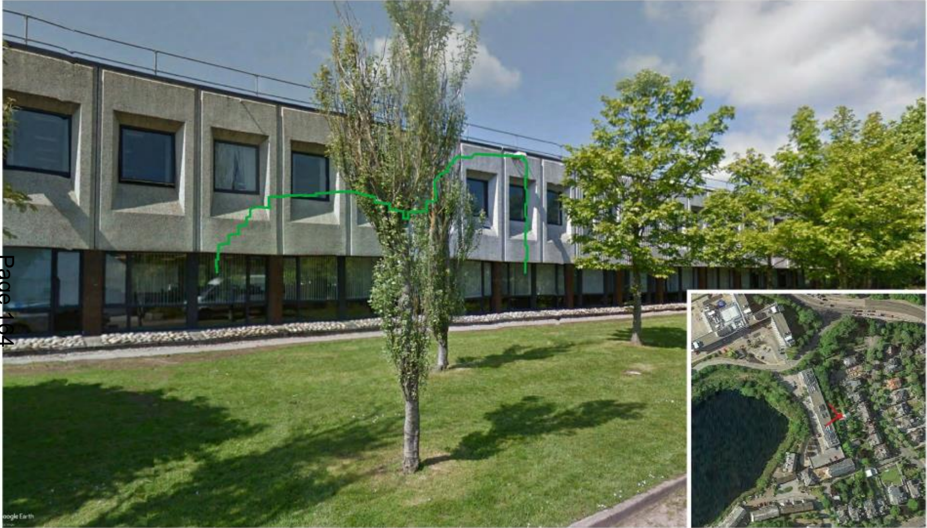
View from Royfold Lane (behind No. 9 Royfold Crescent)
